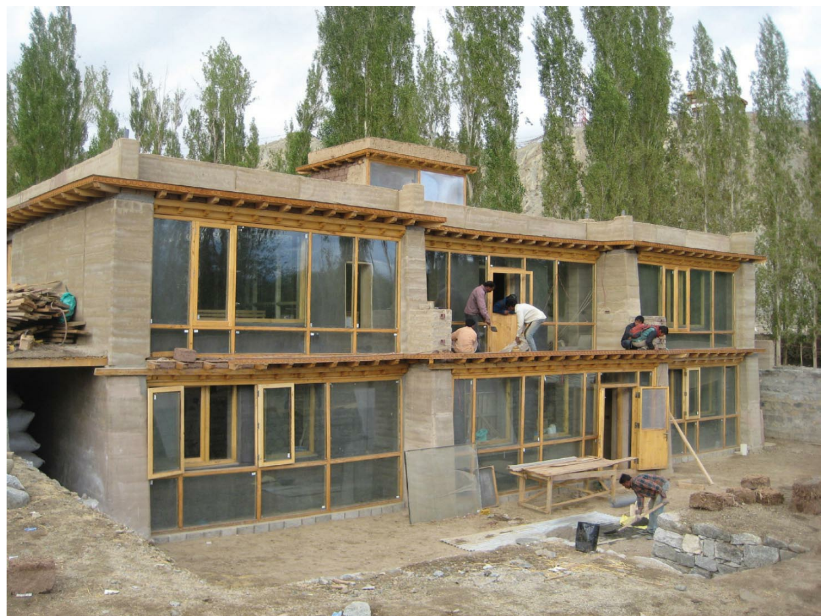
Building a Trombe Wall, a solar efficient wall, using simple means.
